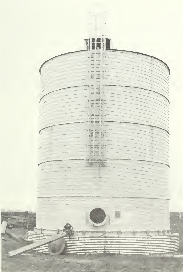
Figure 6.2.13 A cable-wrapped, fiberglass-reinforced grain bin. Arkell Research Station, Ontario Ministry of Agriculture and Food, Guelph, Ontario.
